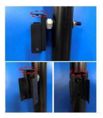
2. Hang the device and tighten the screws (three, the screws are in the device box)
